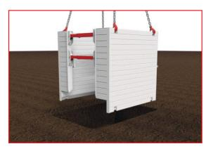
**2:** Lift the Manhole Box into the starter hole.
