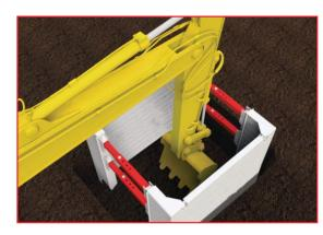
**4:** Excavate beneath the panel and remove any excess material.
